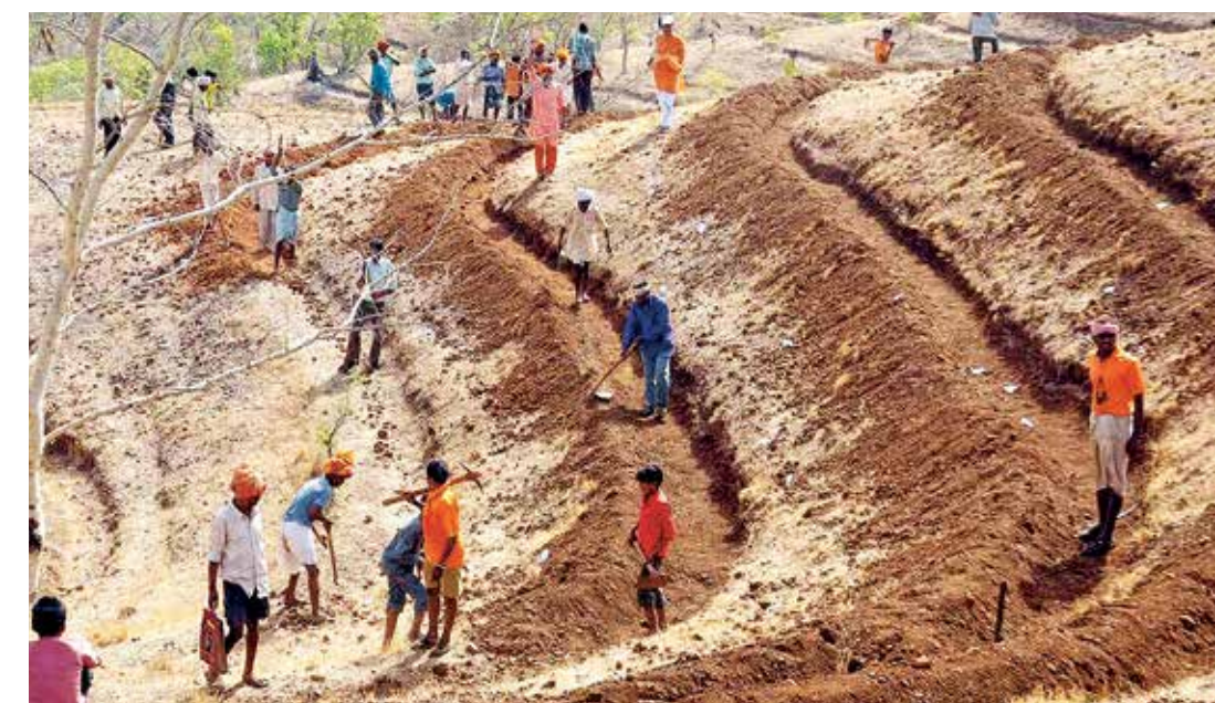
Contour trenches are built to capture the rain
