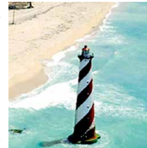
After the tsunami, the lighthouse stands in the sea
