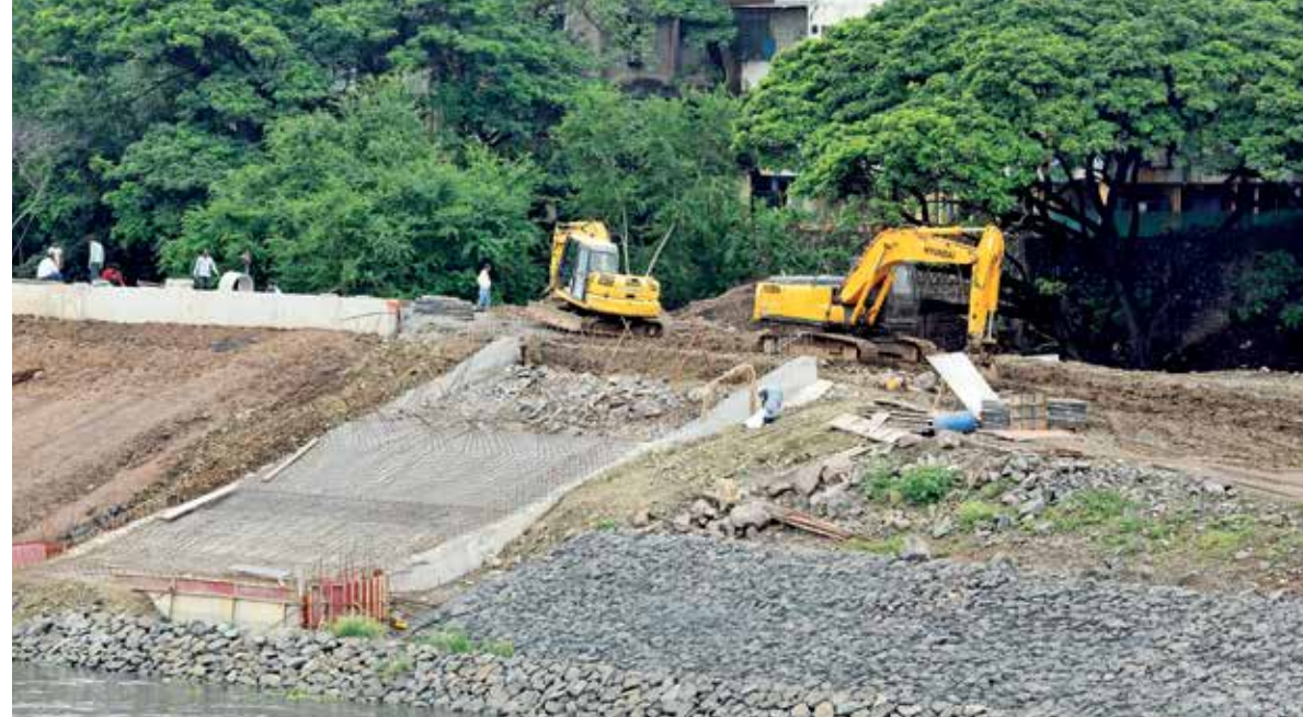
Earthmovers at work on the bank of the river
