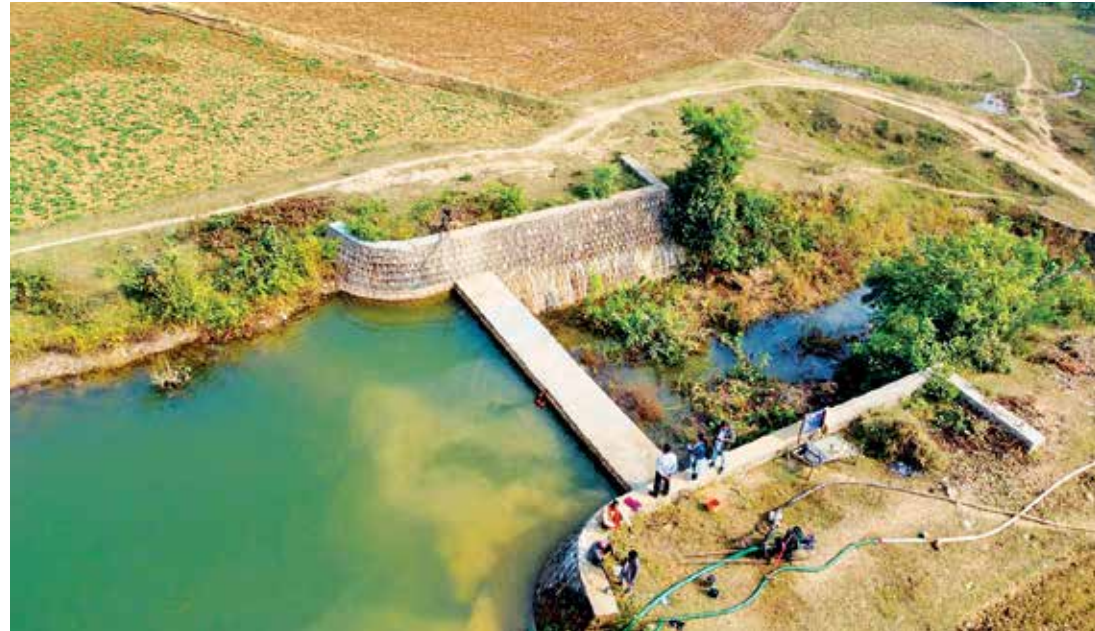
A check dam is repaired in Goiya Khurd village
