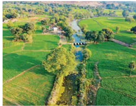
The nullah was also desilted
