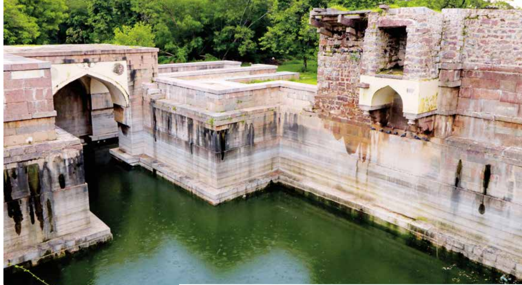
The Idgah Baoli brimming with water after restoration
