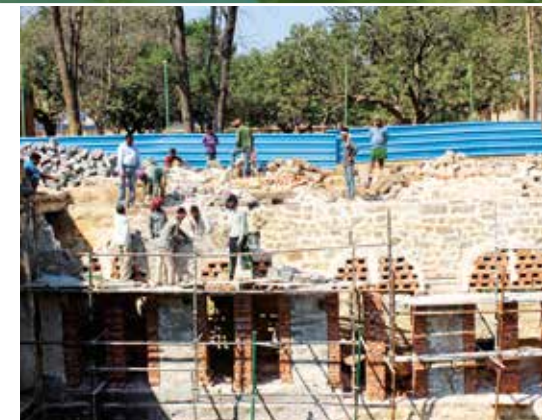
Restoration work in progress
