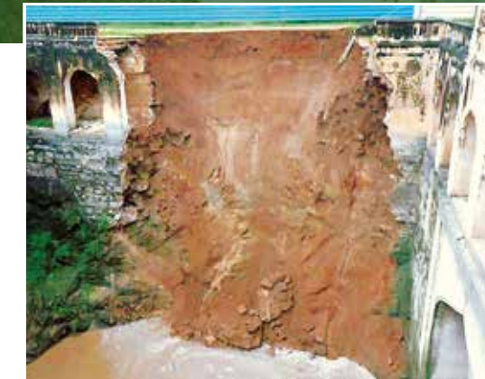
The collapsed state in which the Badi Baoli was found
