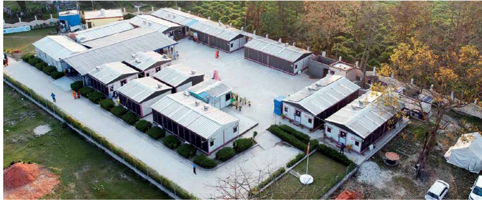
An aerial view of the prefabricated structures of the hospital
