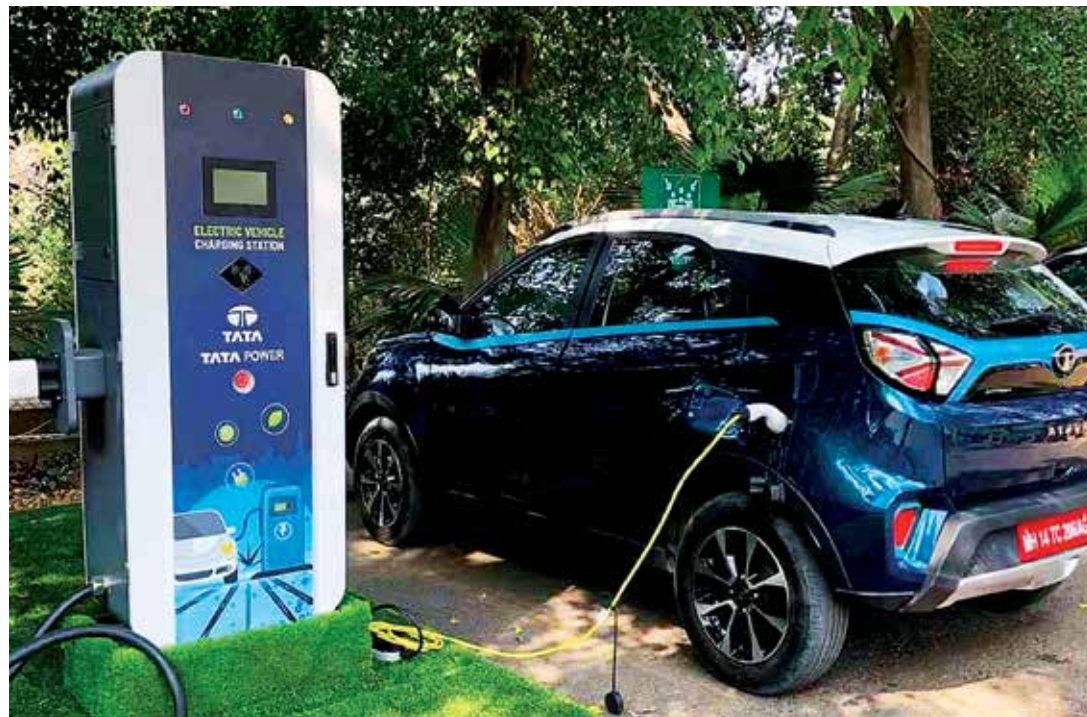
Tata Power's EV app shows you the nearest charging stations
