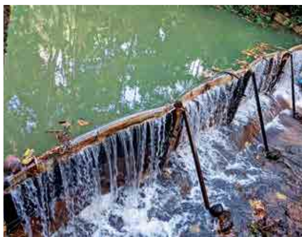
The check dams are stable and can withstand surprise showers
