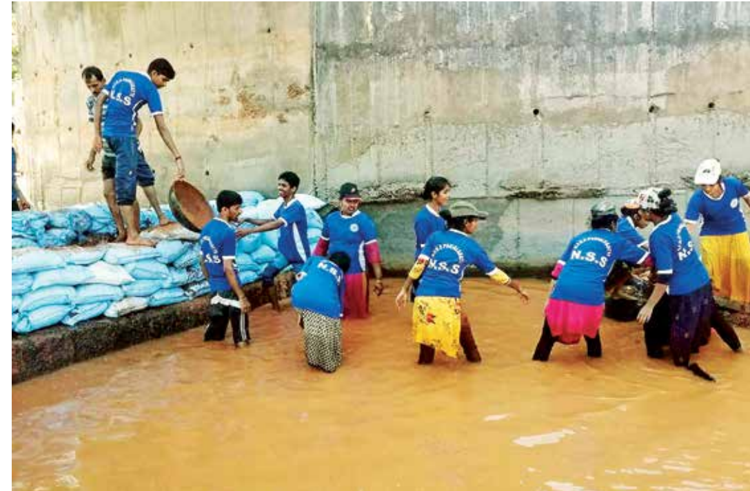
College students pass on sand bags to put in place a check dam
