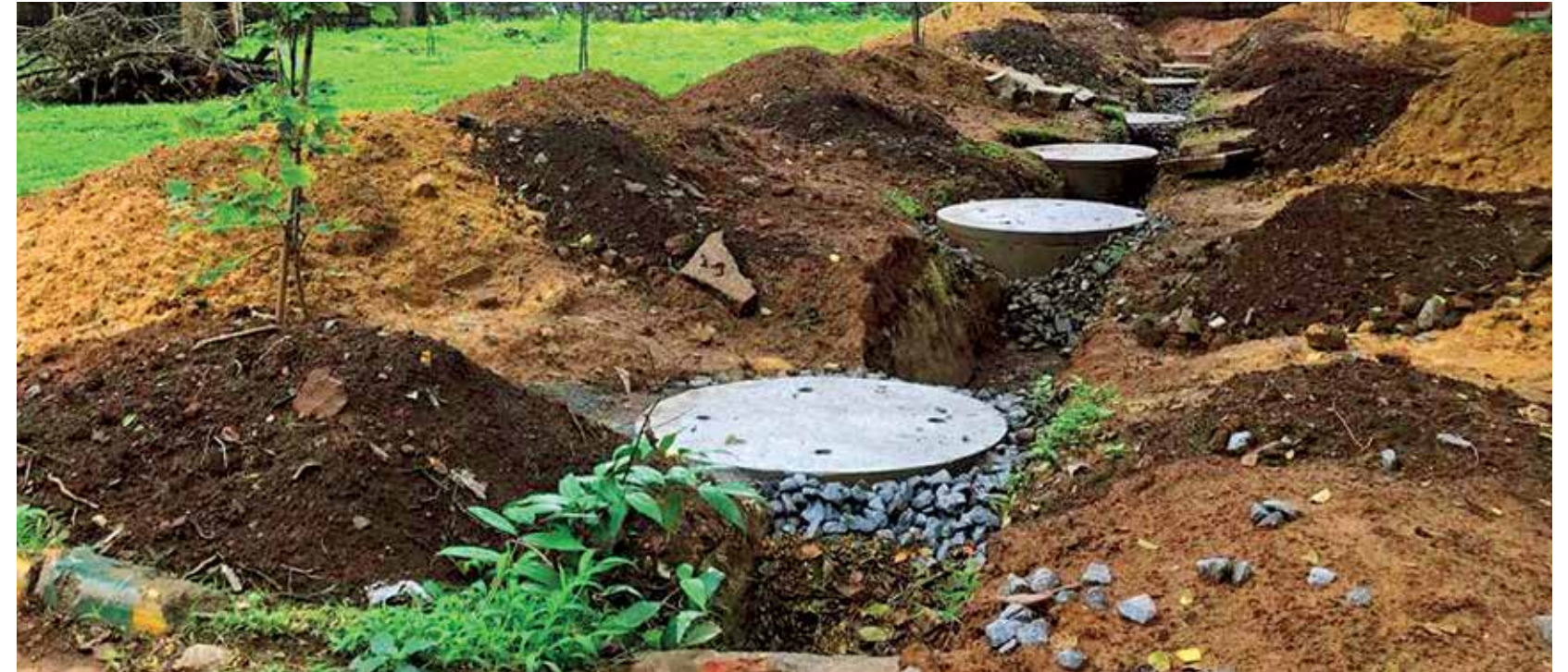
A row of recharge wells at Lalbagh in Bengaluru
