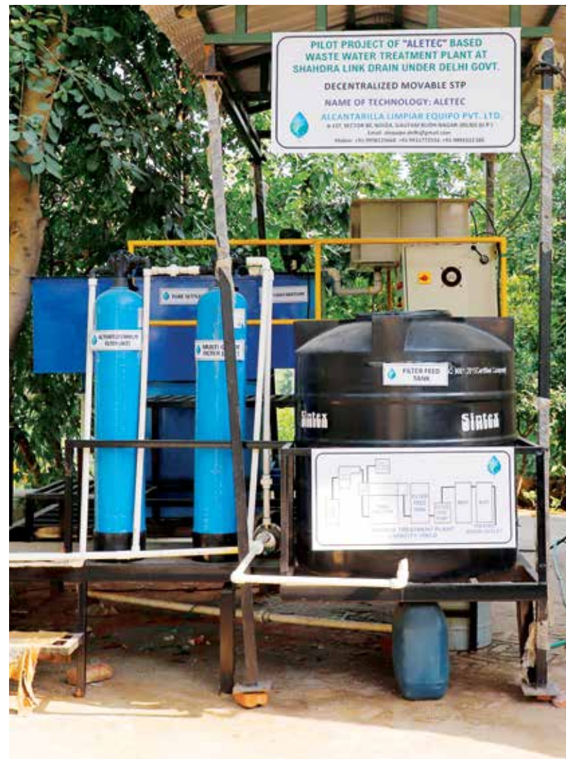
The electrocoagulation unit occupies just nine square metres
