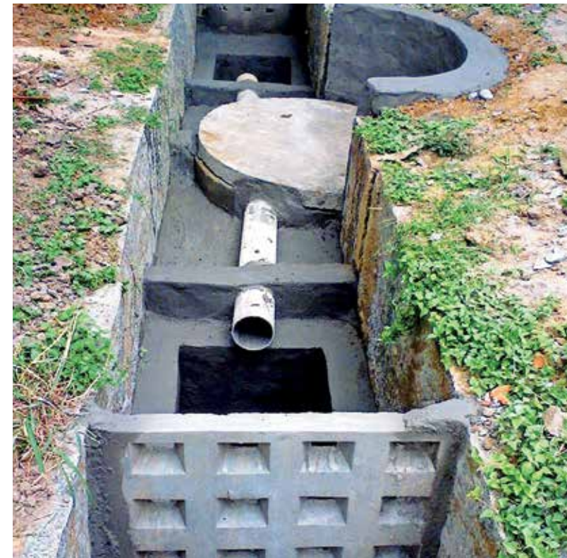
Recharge wells dug in a stormwater drain at Rainbow Drive
