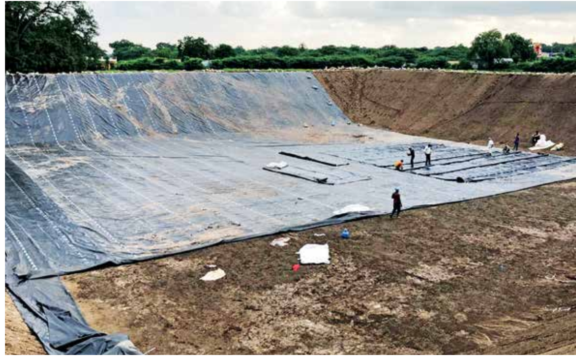
Yogiraj Kolhar uses this tank lined with a plastic sheet to store water for his grape garden in Tikota in Bijapur
