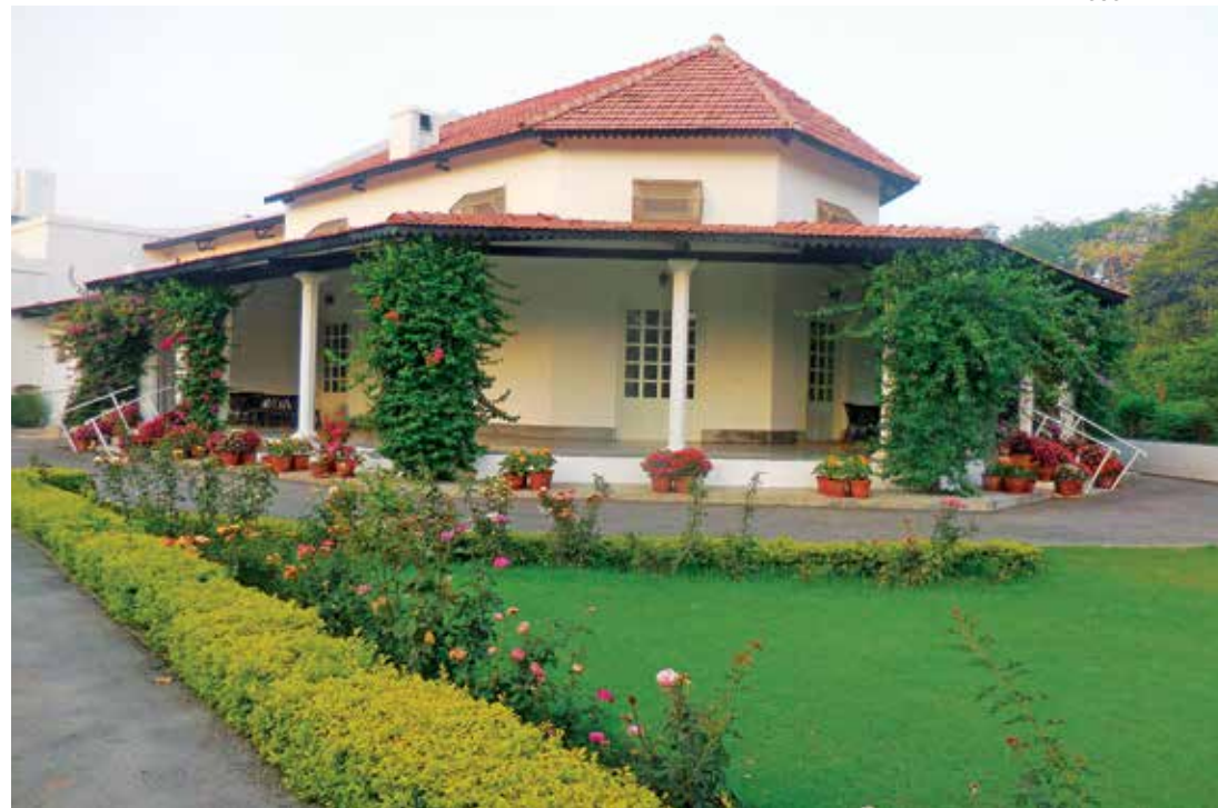
The Obeetee bungalow is a heritage structure
