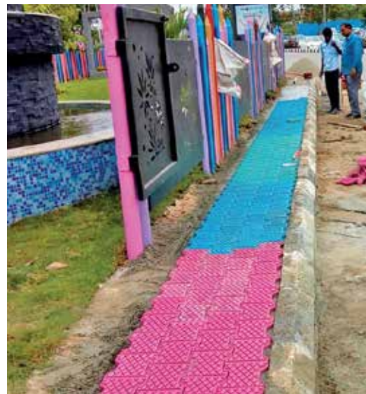
A pavement being built with plastic tiles
