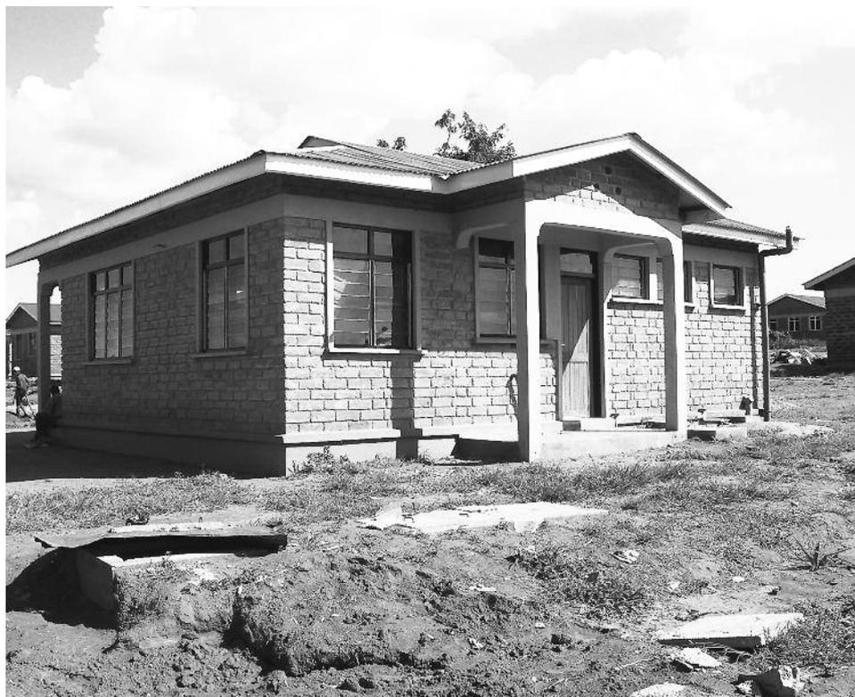
House built using bricks fired in an MRHP-designed kiln in Tanzania.
