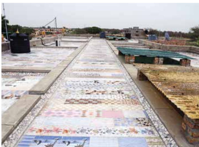
Fixing the leaky roof was crucial. Now it is properly tiled
