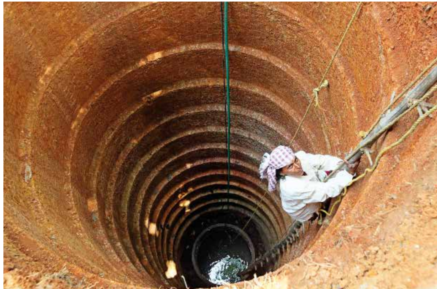
The women have learnt to build wells with circular steps. The quality of their work is as good as professional male well diggers
