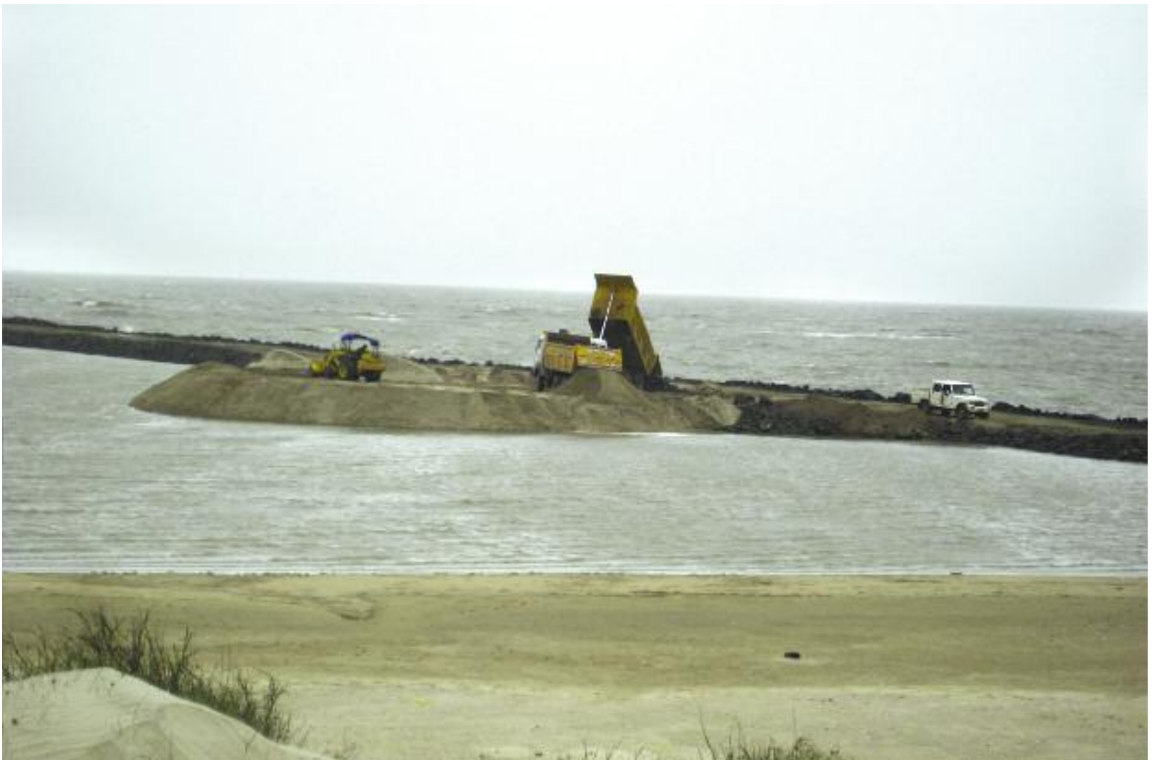
Dredging activity at the Mundra Port and SEZ Ltd
