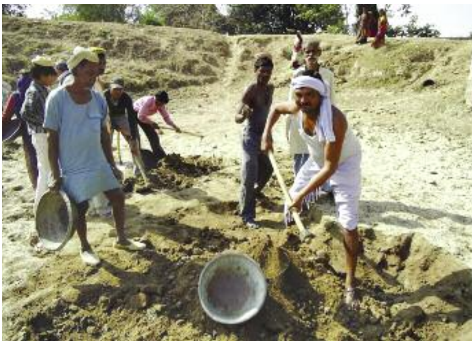
Lalaram at a work site
