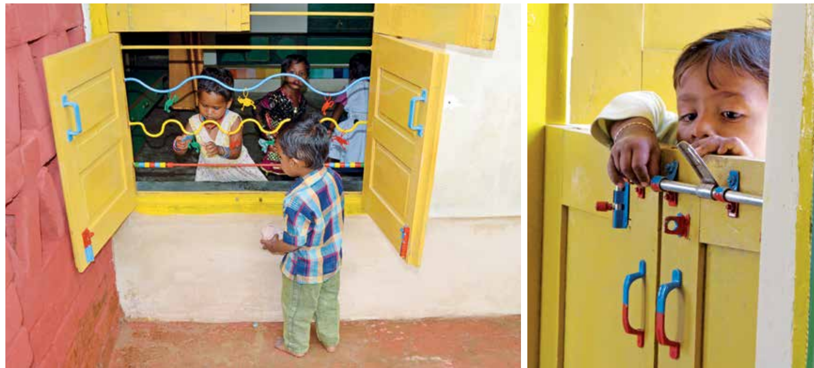
Lowering windows and using grills creatively makes a huge difference
