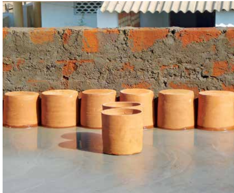
Inverted pots on a roof used as thermal insulation to keep the indoors cool in Chhattisgarh
