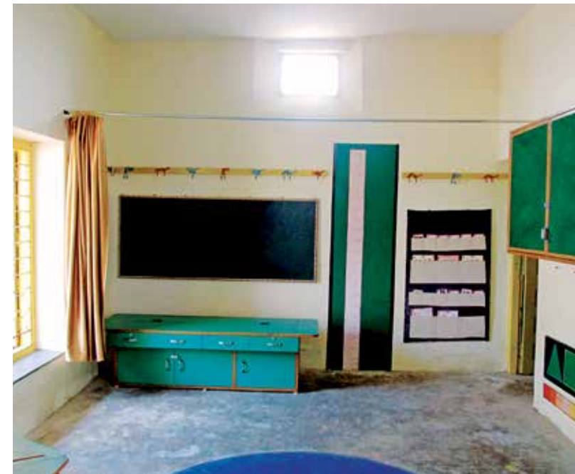
Ventilators serve to bring in more light and fresh air like this one in an activity room
