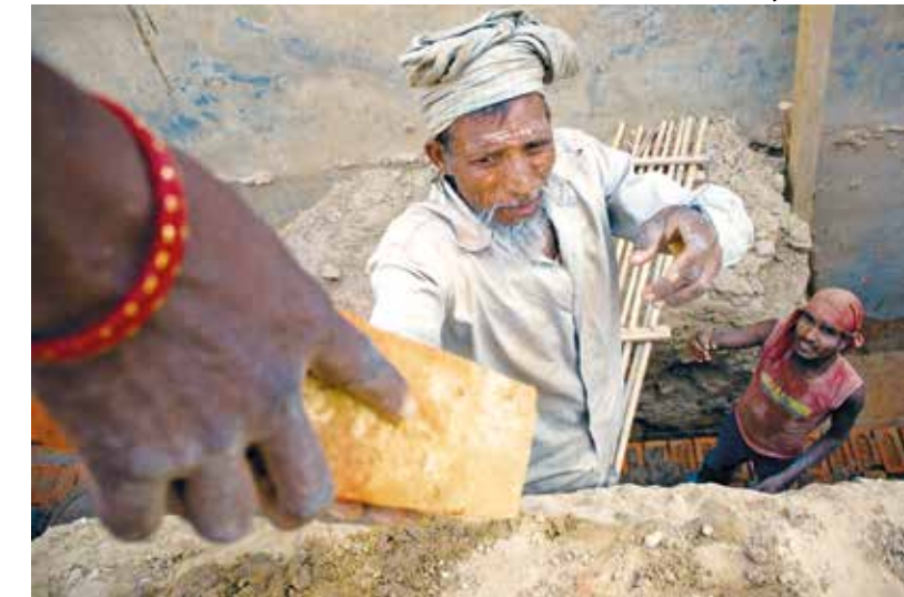
Workers pass bricks at a site in Gurugram
