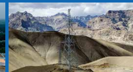
India's highest Transmission Line (13,500 feet)
