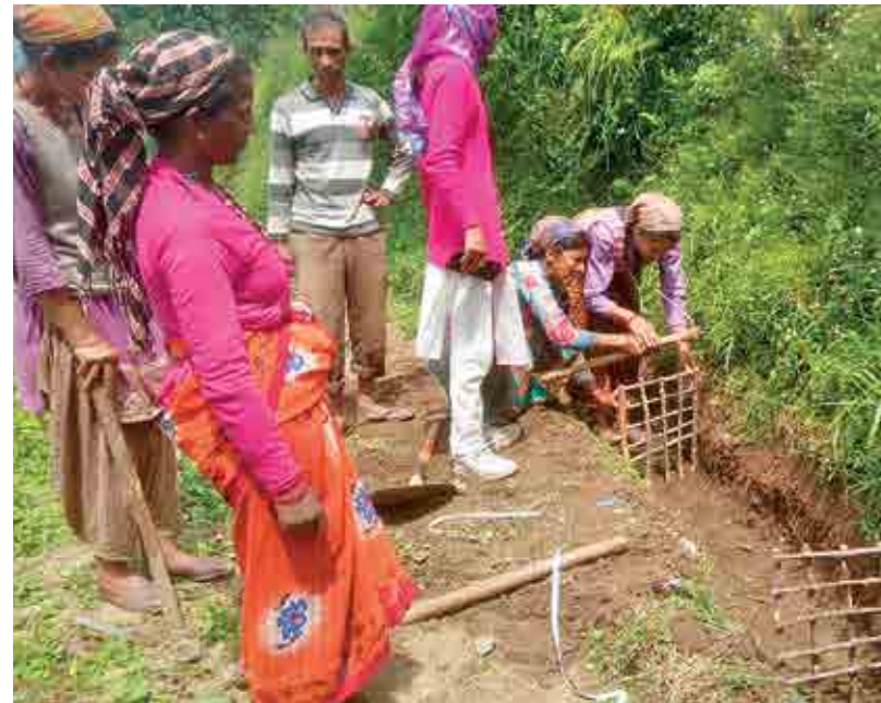
A trench being dug in a recharge area
