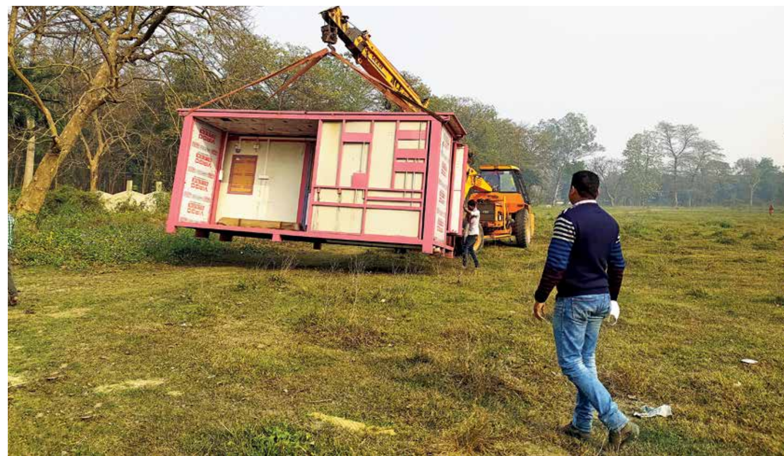
A cabin being hauled by a crane
