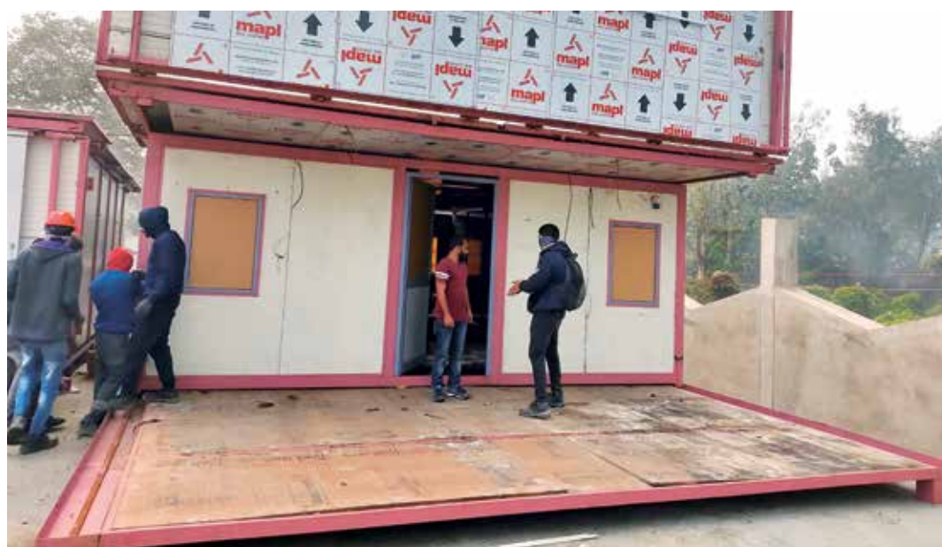
A part of the hospital erected and awaiting finishing
