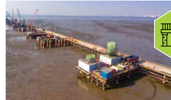
Constructing 7.8 kms long bridge section of Mumbai Trans Harbour Sea-link Project
