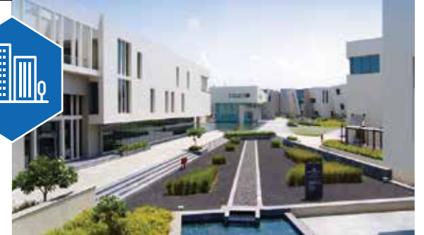
An IT Park of 1.0 Mn Sq. Ft. BUA, spread across 100 acres constructed in Indore
