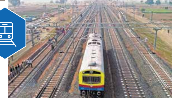
Successfully completed LOT 102 and 103 of Dedicated Freight Corridor Project
