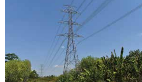
Completed 41.42-km Transmission Line Project of 500kV in Thailand
