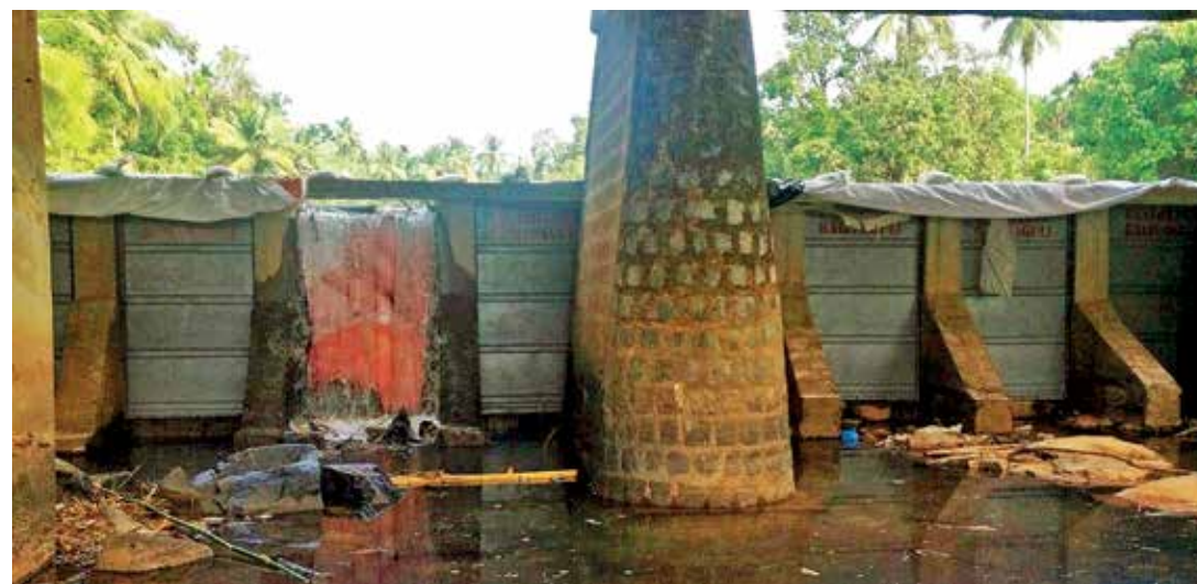
The abandoned bridge was creatively used
