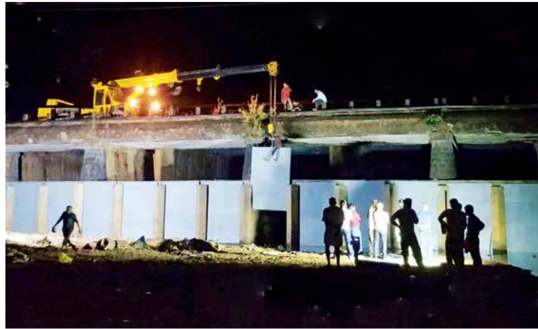
A crane on the bridge placing the shutters on the dam
