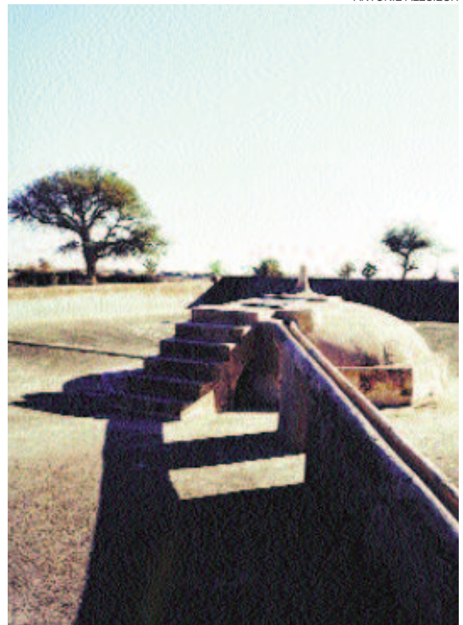
Kund at Sikar. The channel leading out provides water to animals and people. This prevents people from entering all the time and contaminating the Kund's supply.
