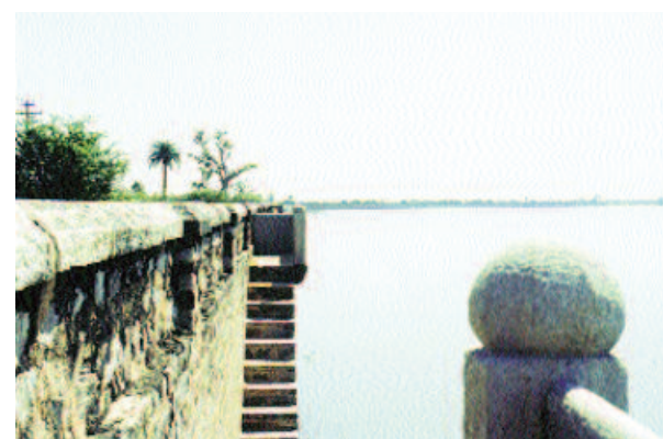
The Toda Rai Singh tank was built at least 350 years ago to serve the irrigation needs of 18 villages. Incredibly, it still performs that role though it has been acquired by the irrigation department of Rajasthan.
