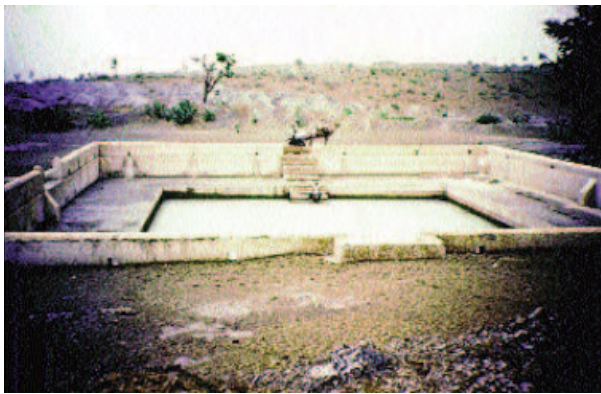
A Johad in Churu district, a marvel of engineering. It has three tiers on four sides. The structure is designed to reduce evaporation. Narrow ledges trap silt.
