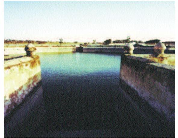
A hexagonal Johad with embankments built 200 years ago to catch the rain and ensure a local supply of sweet water. A modern water plant lies derelict on its periphery.
