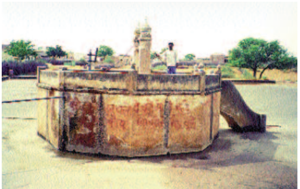
A Kund in Taranagar, district Churu. Rain that falls on the surface of the Kund goes through tiny filters to collect 40 feet below. The area is saline.
