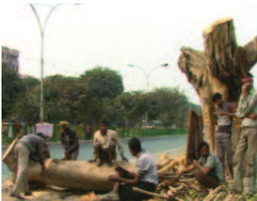
Trees are being chopped for concrete
