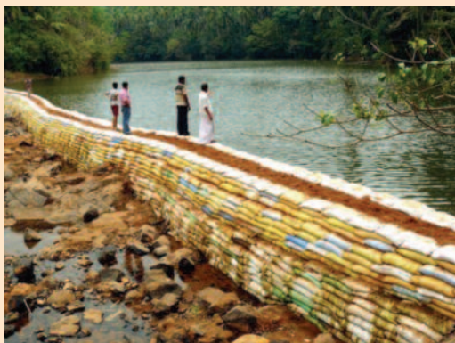
Check dam made with sand in plastic bags
