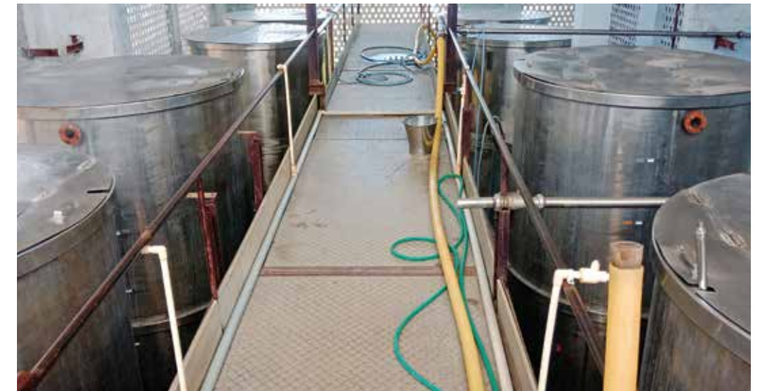
The microbrewery is modern and well-designed
