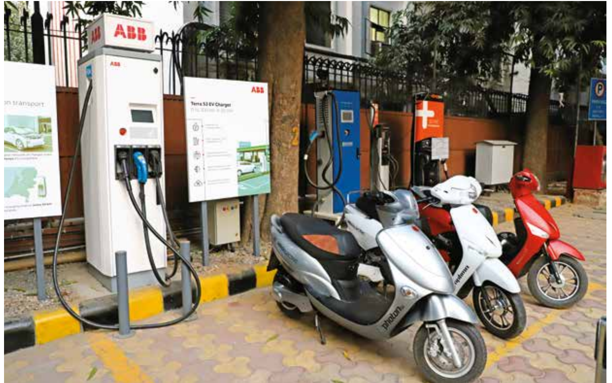
A charging point at NITI Aayog's office: The government's renewable energy target has come as a boost
