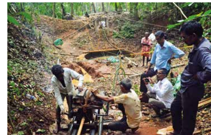
The ada bore taps water only from shallow aquifers
