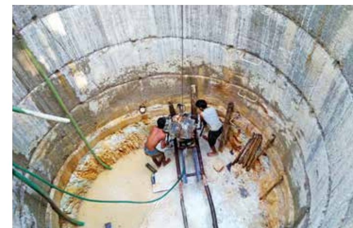
Most horizontal wells are dug from inside open wells
