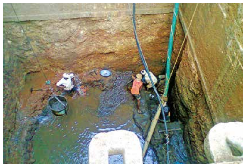
The Barah Gade well being desilted and cleaned
