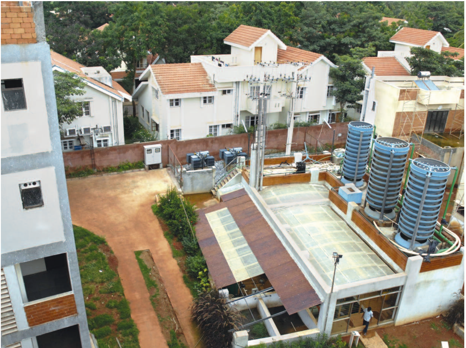
BCIL's housing colonies aspire to be self-sustaining and are innovative in their use of technology
