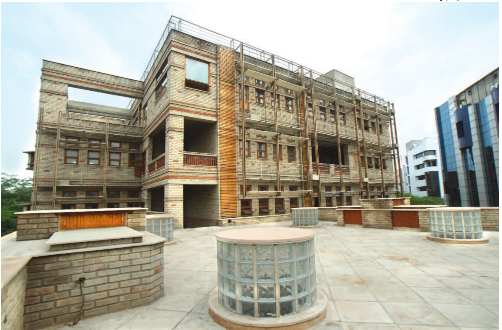
The Development Alternatives' new office building
