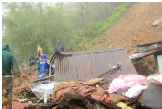
House crumbles under landslide
