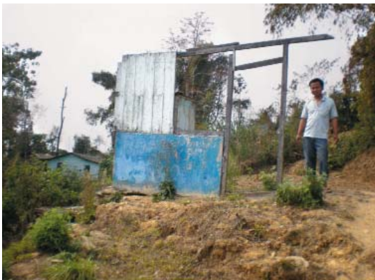
Landslide- hit home
