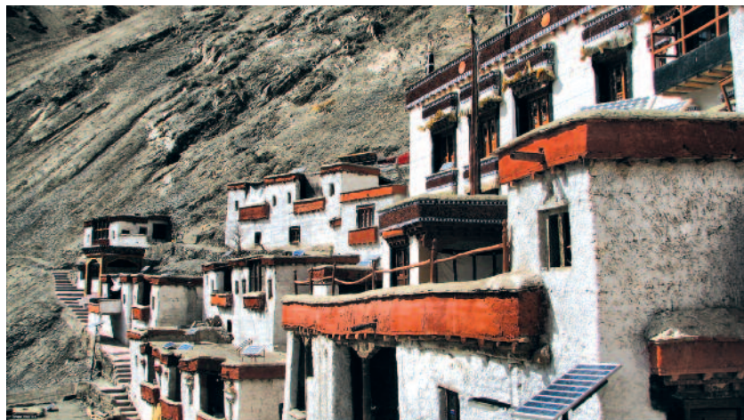
Unused to raindrops hammering down, Ladakhi homes collapse.
