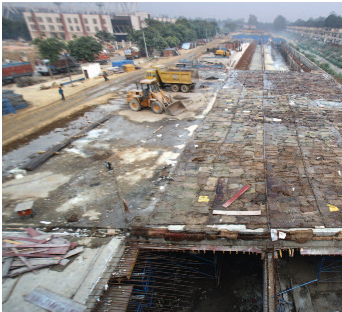
Stretch of a nullah being covered up to make a parking lot for the Commonwealth Games
