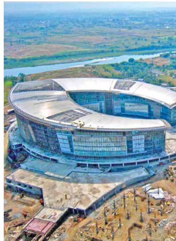
An SEZ being constructed. India has over 500 SEZs.
