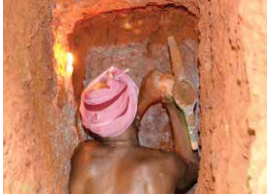
Kunhambu digging a suranga
