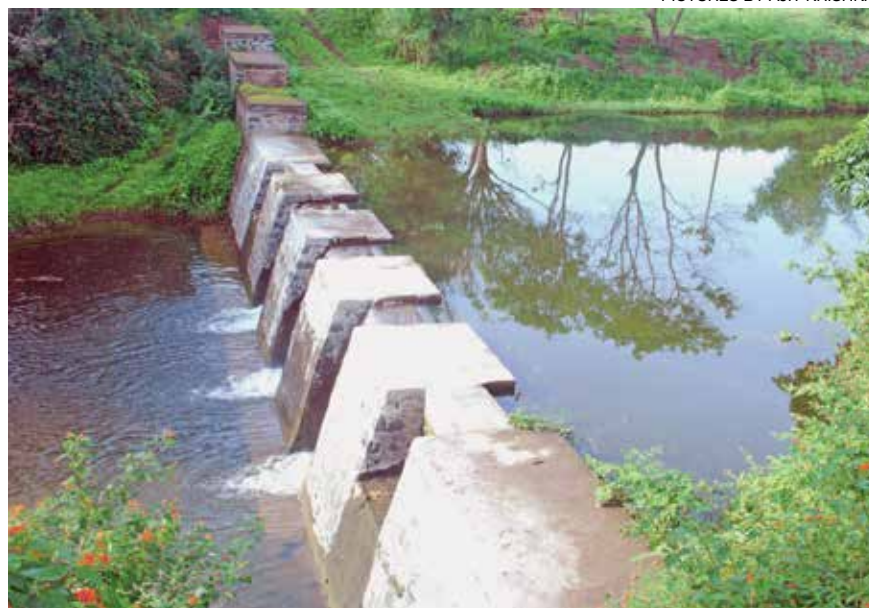
The revived KT Bandhara dam in Jakhangaon
