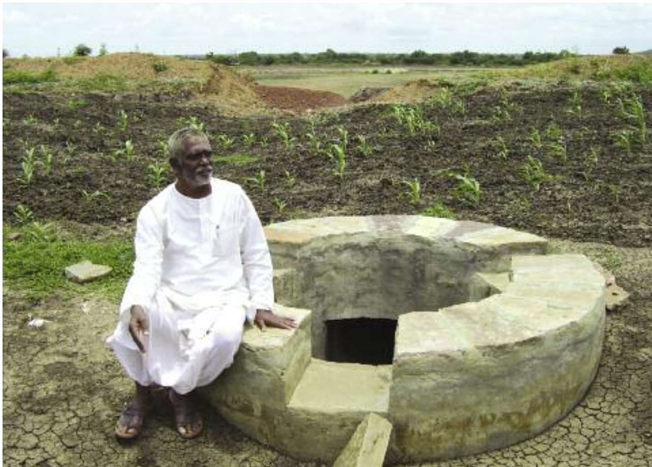
Mallanna Nagaral near a drop inlet spillway. Run-off from the upper fields will bring topsoil and fill the land around this structure.
