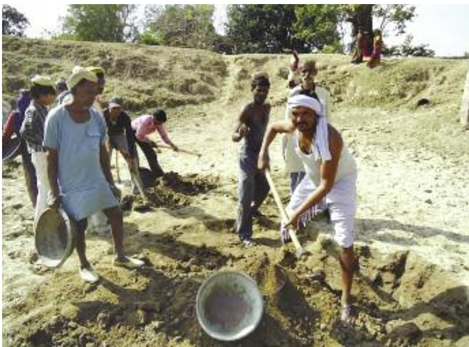
Lalaram at a work site
