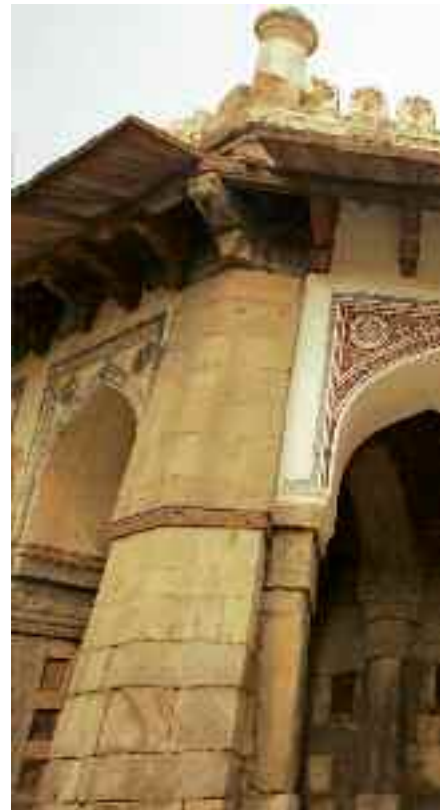
The restored facade of Isa Khan's tomb
