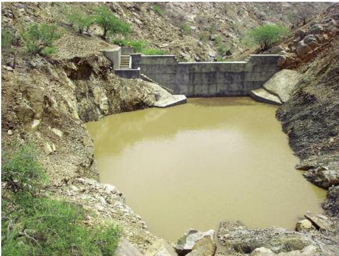
The check dam on a hilltop which was built for Korsina
