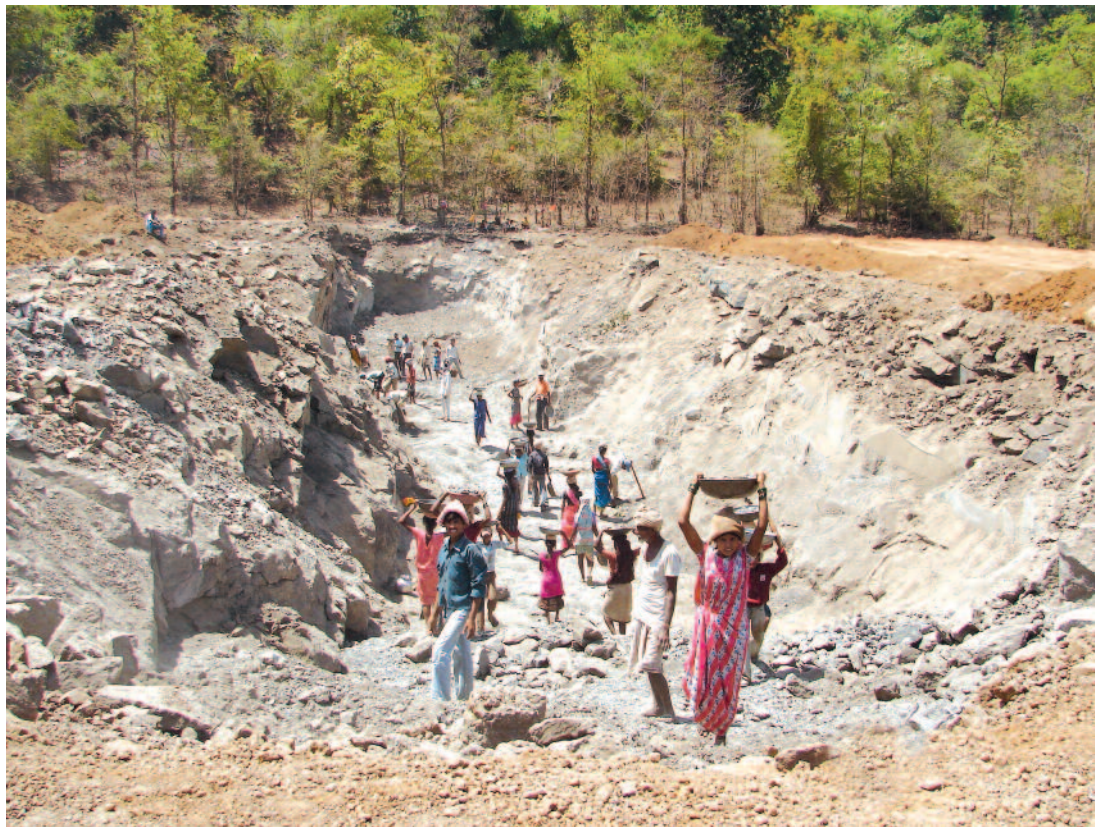
A dam being dug in Maharashtra
