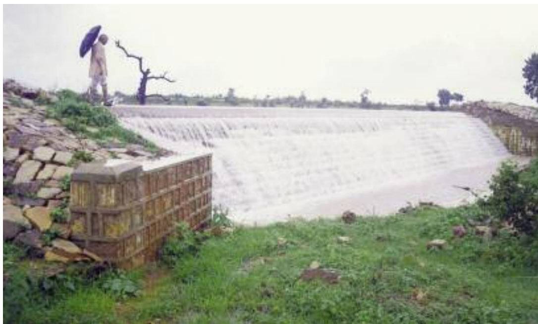
Check dam built by the ABSSS
