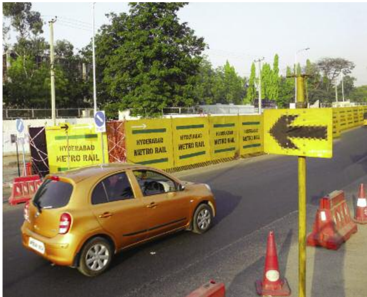
Work in progress, but is it enough?
