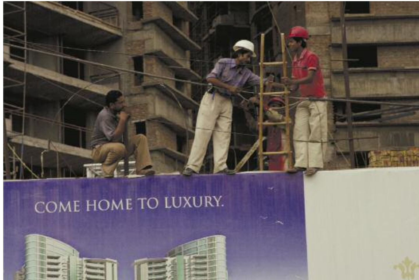
Doom or boom? Construction workers at a site in Gurgaon
